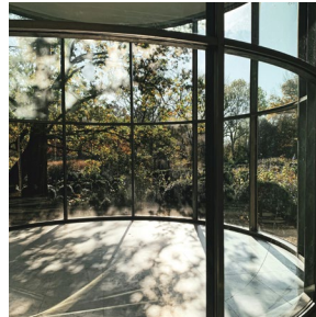
Fixed partitions & glass walls
